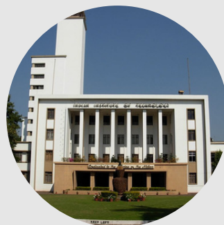
Indian Institute of Technology, Kharagpur Electrical Engineering
